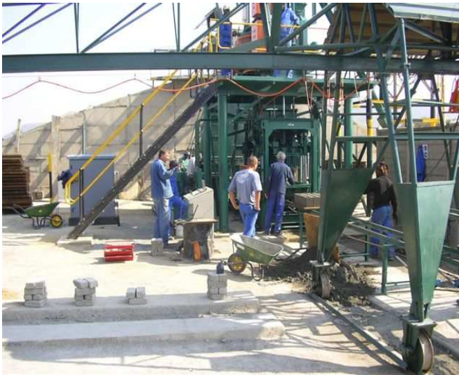
The new VB 4 plant under construction
